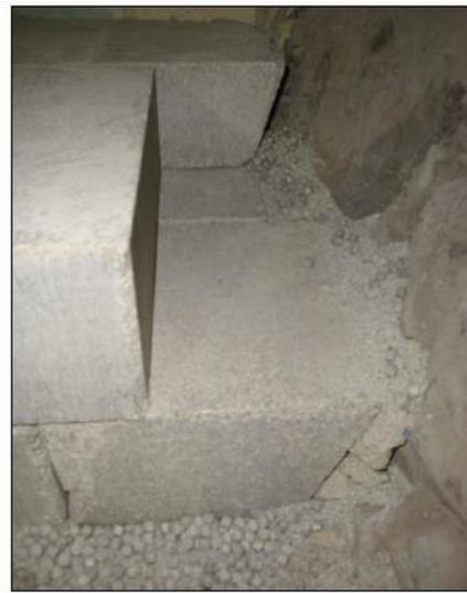
**Figure 4** Installation of bentonite core, wall made with bricks, pellets/powder mixture between claystone and bentonite bricks. Background: hydration membrane
