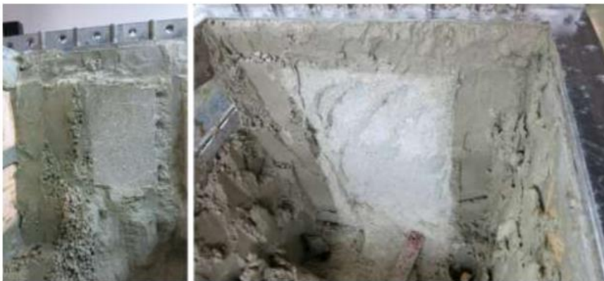
Figure 2. Cross sections from the tunnel during the dismantling. There were 6 backfill blocks in the tunnel surrounded by a backfill pellet layer.
